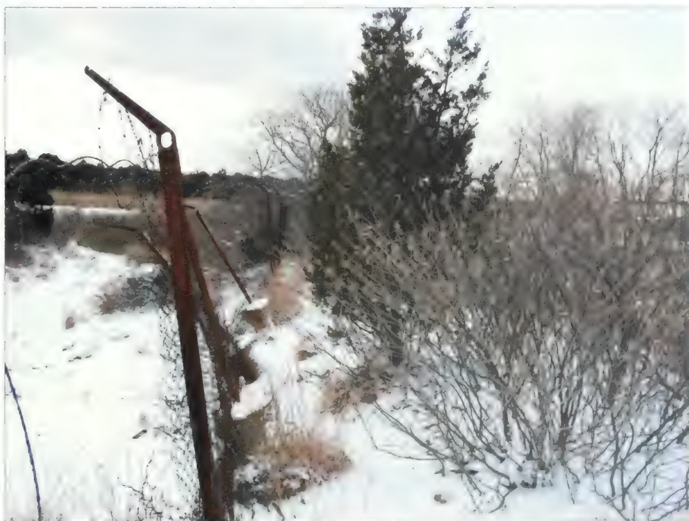
Figure 5.105. Existing perimeter fence, NIKE launch site. The existing perimeter fence at the radar and launch sites should be clearly delineated and maintained by removing all woody vegetation a minimum of four-feet off either side of the fence. The vegetation removals will also aid in inspection and repairs of the existing fence (Olmsted Center, January 2009).
